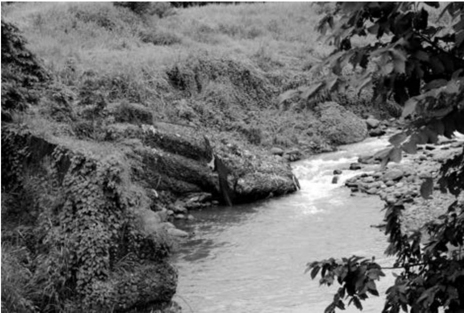
One of the gabions that fell after the first rains, August 2022.
